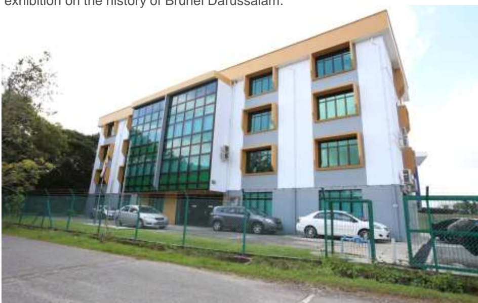
THE BORNEO RESEARCH CENTRE BUILDING IN ANGGEREK DESA
